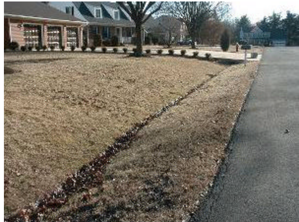
Developers can eliminate curbs and gutters to disconnect impervious surfaces and promote infiltration of storm water on vegetated areas (such as this grass-lined channel in a residential neighborhood)
