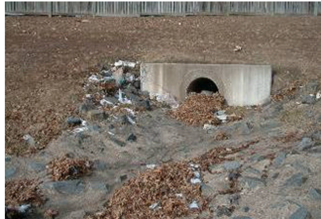
Regular inspection and maintenance of storm water best management practices is important to ensure that the practices are functioning properly and to remove trash and organic debris
