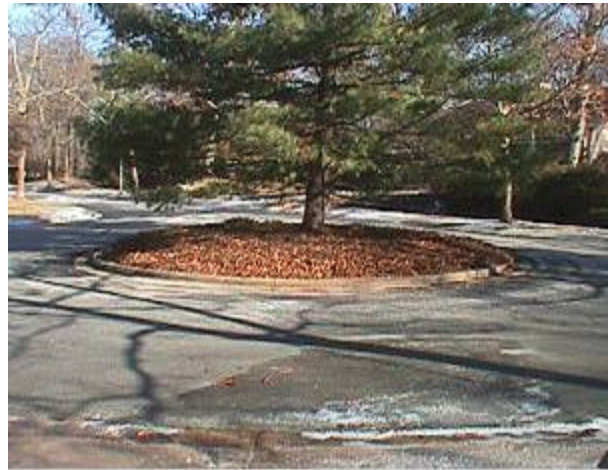
Rather than having a fully paved cul-de-sac bulb, site designers can incorporate pervious circles with vegetation that reduce the site's overall impervious area
